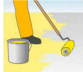
Even application of Primer coat Sikafloor®-156 / -161 and the conductive Layer Sikafloor®-220 W Conductive : with medium to long haired roller or brush. E.g. Polyplan roller and brush.
