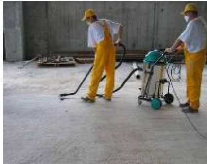
Cleaning of the surface
