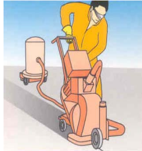
Preparation of the substrate: Blast cleaning or other mechanical means e.g. Blastrac
