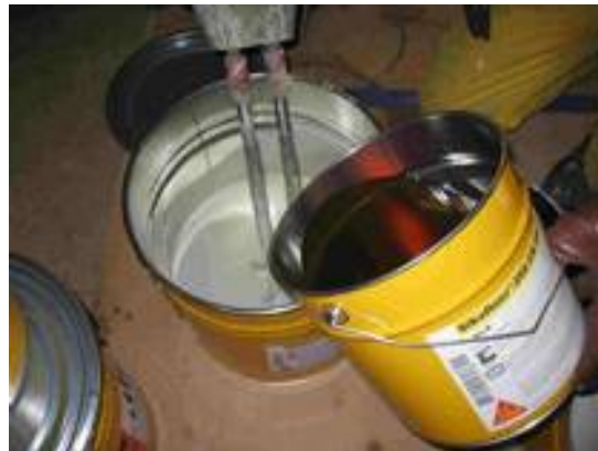
Mixing of Sikafloor®-262 AS N
