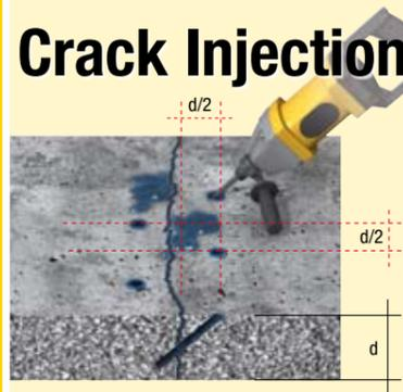
1. Drill packer holes at a 45° angle to the concrete surface as shown in the figure.
