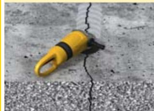
1. Prepare the substrate by blast cleaning or mechanically by grinding etc., then clean by brush and vacuum.
