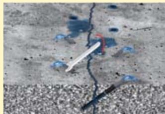
2. Install the mechanical packers. Tighten the mechanical packers so that they can withstand the maximum injection pressure.
