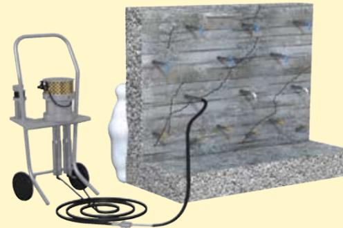
4. When the injection material flows out of the second packer during the injection process, fix the non-return valve on it as quickly as possible. Stop injection at the first packer and continue at the second packer.
