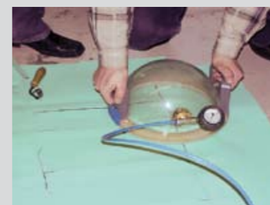
■ Secure and homogeneous with welded seams tested on site
