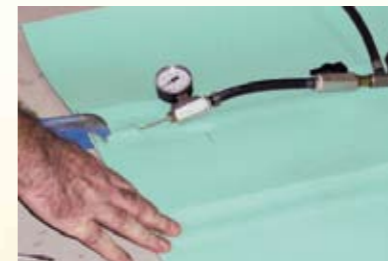
Physical testing of double welded seams and central void with compressed air
