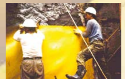
Ignoring substrate requirements and omitting protective backing materials
