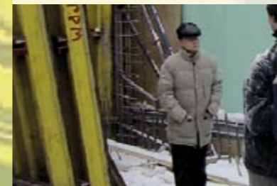
Membrane installation at extremely low temperatures
