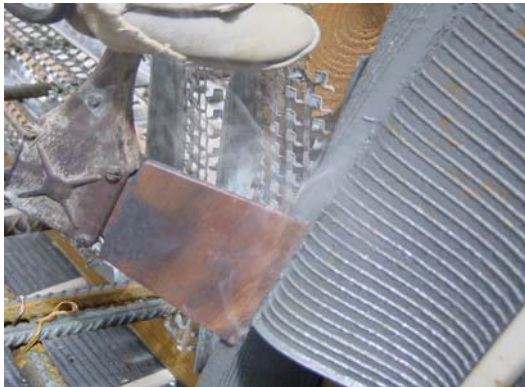
2. Overlap welding using electric “axe”
