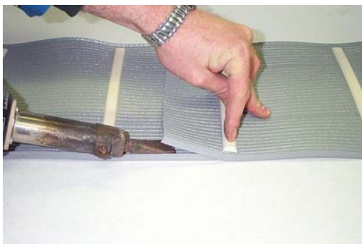
3. Overlap welding using hot air welder
