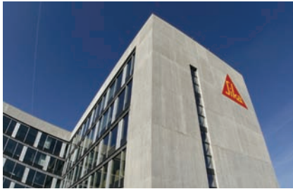
Fig. 8.12.2: With a wide variety of formwork and treatments available, almost any concrete finish can be created, included mirror smooth, plain timber board or other patterns, bush hammered or exposed aggregate etc..
