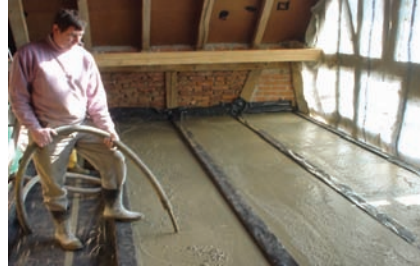
Fig. 8.15.1: The compressive strengths obtainable are always linked to the existing density of the materials. The level of this correlation can be altered through the quality of the aggregates. As can be expected, voids result in very low strength and so-called expanded clays can also give very good strength development at low densities of around 1'500 kg/m 3 .
