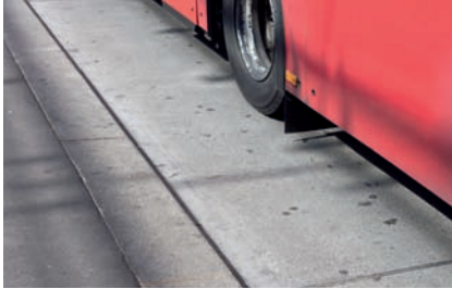
Fig. 8.7.3: Concrete roadways and other publicly accessible areas, especially those experiencing high volumes of traffic or concentrated loads, are subject alongside high mechanical burdens also to strong abrasion, often presenting the risk of a smooth, slick surface.
