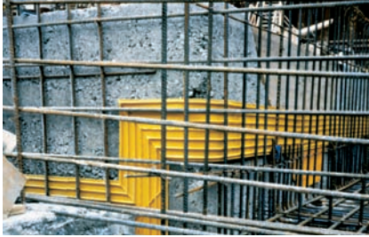
Fig. 8.1.2: Sika waterbars are flexible preformed PVC waterstops for the waterproofing of both movement and construction joints which can be subjected to low and high water pressure.
