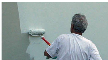
Fig. 8.8.2: As resistance of concrete against chemical attack is limited, protective coatings are a often used external protection. Epoxy resin-based protective coatings are applied over the entire surface following reprofiling of the concrete surface with sulfate-resistant repair mortar enhanced with synthetic material.
