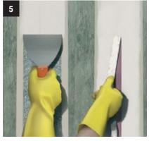
Apply the **Sikadur<sup>®</sup>-Combiflex<sup>®</sup> CF** adhesive on the left-hand and the right-hand side of the joint. Then remove masking strip.
