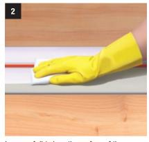
In case of dirt clean the surface of the **Sikadur-Combiflex**<sup>®</sup> **SG** tape with a dry or wet cloth. Use water and **no solvent** for cleaning.
