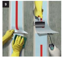
Connect tape ends by hot air welding. **Prepare the welding area by roughing the surface by scotch brite or sand paper.** Overlap 40 - 50 mm.
