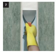
Apply the **Sikadur<sup>®</sup>-Combiflex<sup>®</sup> CF** Adhesive on the tape.
