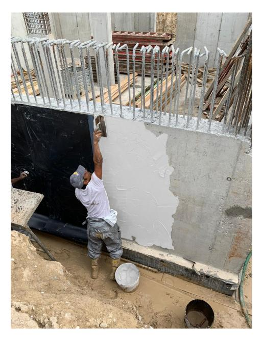
**The self-priming cement-based adhesive, SikaShield® W1,** acts as levelling compound and a sealing adhesive resulting in a strong and lasting bond between the concrete substrate and the membrane, avoiding any lateral water migration and reducing the risks of leakages.
