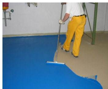
Sikafloor®-264 applied as a seal coat by squeegee.
