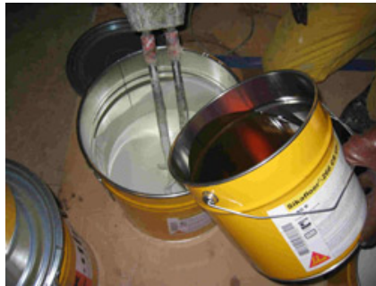
Mixing of Sikafloor-264.
