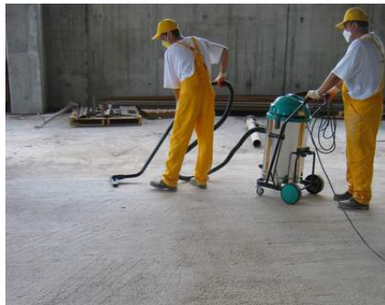
Cleaning of the surface
