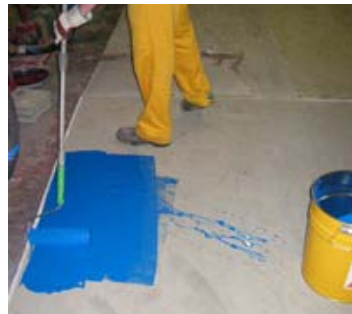
Sikafloor®-264 applied as a coating.
