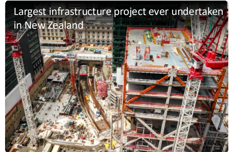
City Rail Link, Auckland, New Zealand
