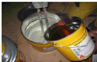
Mixing of Sikafloor-263 SL.
