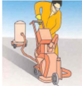
Preparation of the substrate: Blast cleaning or other mechanical means e.g. Blastec
