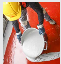
Fig. 7 Pouring the SikaTransfloor®-352 (SL/ST) to the floor
