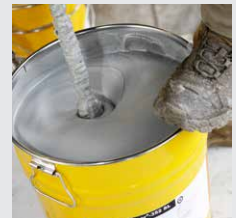
Fig. 5 Mixing SikaTransfloor®-352
