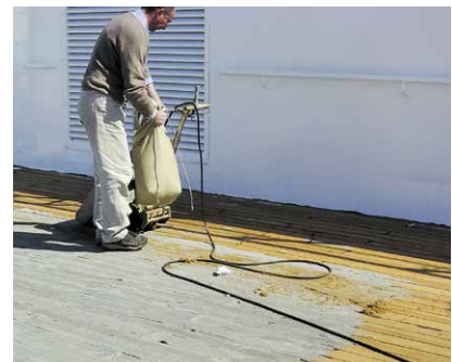
Fig. 20 Sanding the deck
