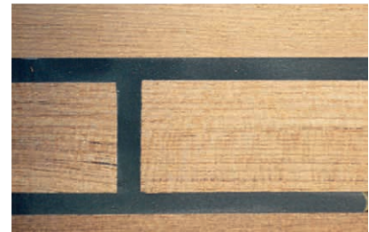
Fig. 29 New teak deck
