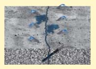
Fix the non-return valve on the first packer and start the injection process.
