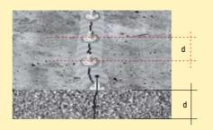
2. Place a steel nail through the packer into the crack to prevent the injection canal from being blocked by the **Sika® Injection-490** adhesive and then install the surface packers as shown in the figure.
