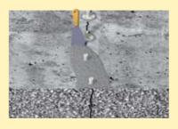
3. Patch the surface of the crack with Sika® Injection-490. Ensure that the packer and the crack on the surface are fully covered by the adhesive filler.
