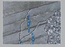
Remedial surface sealing by curtain injection of defects in underground building components.
